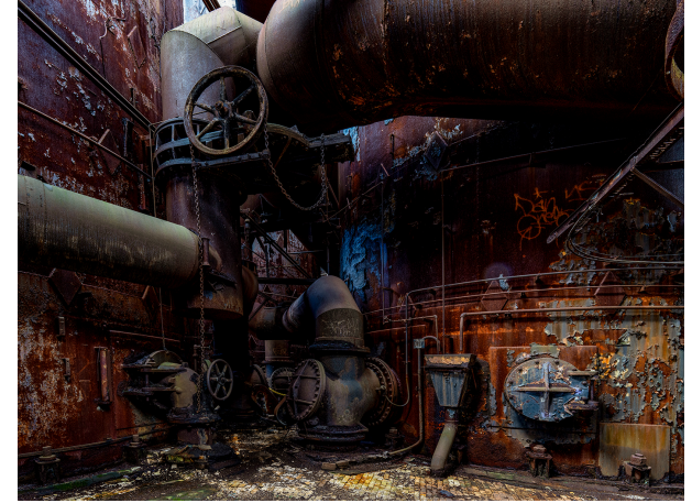
Carrie Furnace Tanks Certificate of Merit Marian Wyse
