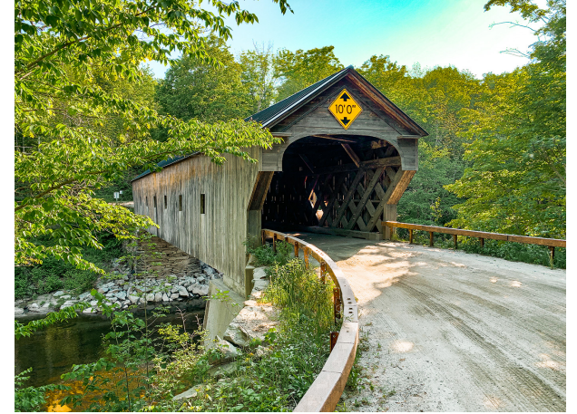
Covered Bridge Vermont Certificate of Merit Daniel Nist
